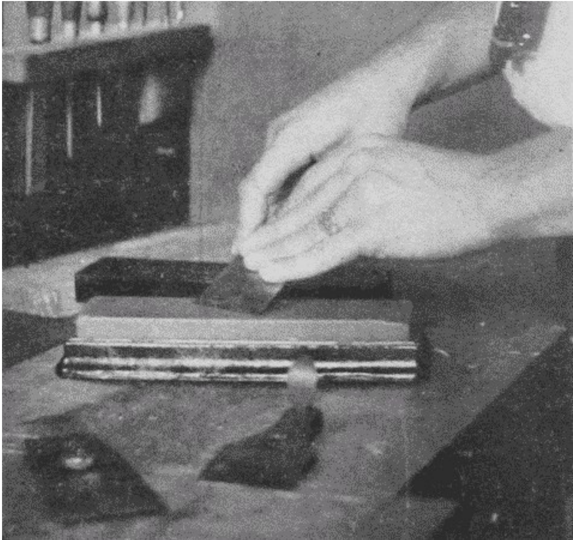
Fig. 77 Whetting a Plane-Bit.
