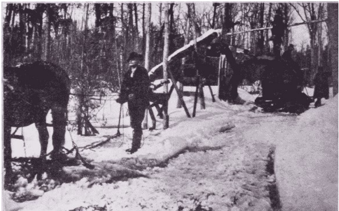
Fig. 10. Making an Ice Road by Flooding.
