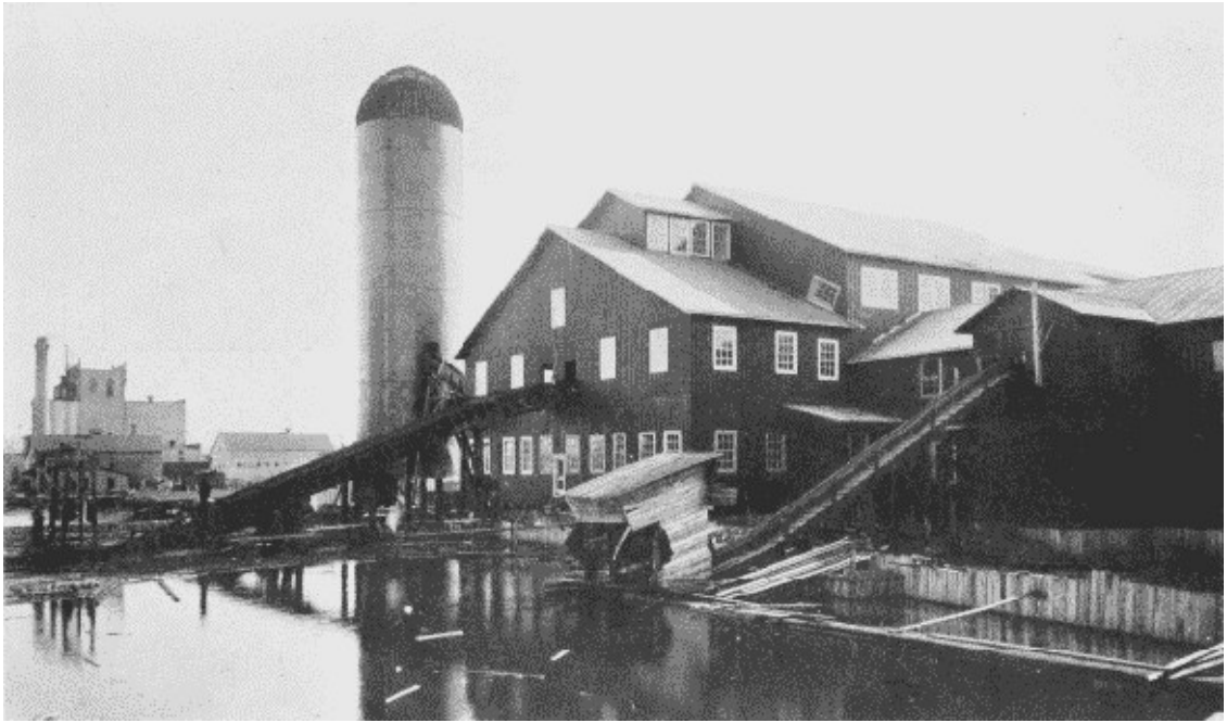
Fig. 37. Two-Story Mill at Virginia, Minnesota, Showing Jack-Ladders and Consumer.
