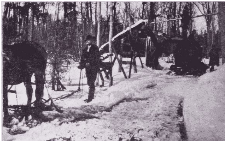
Fig. 10. Making an Ice Road by Flooding.
